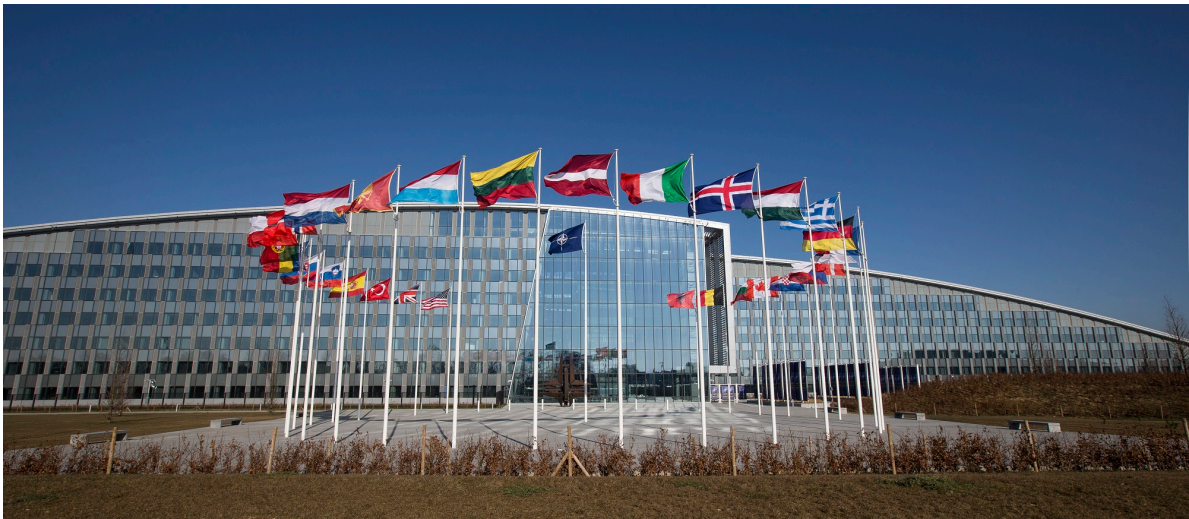
Exterior view of the new NATO headquarters
